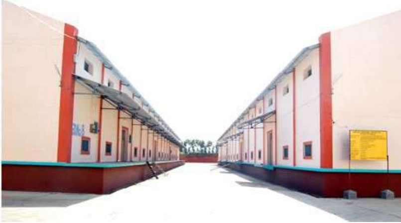
Nanjikottai Warehouse, Thanjavur District.
