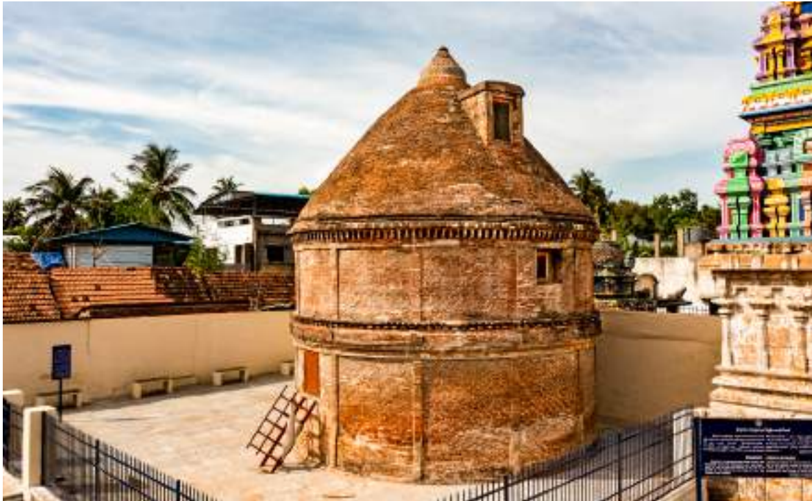
Giant granary, (17 th century CE), Tiruppalaithurai, Thanjavur district.
