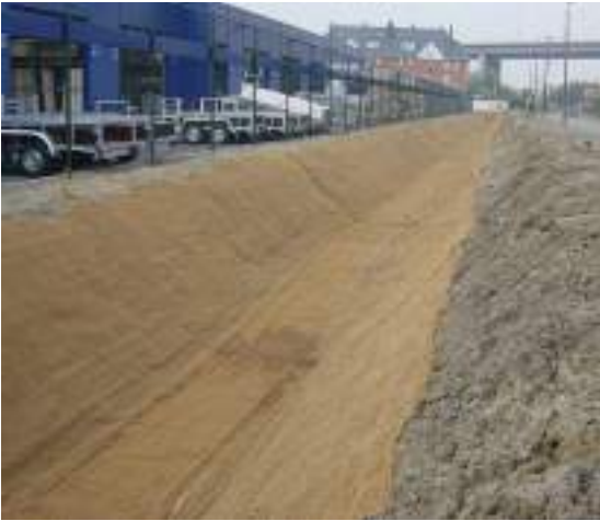
Coir geo-textiles for canal lining
