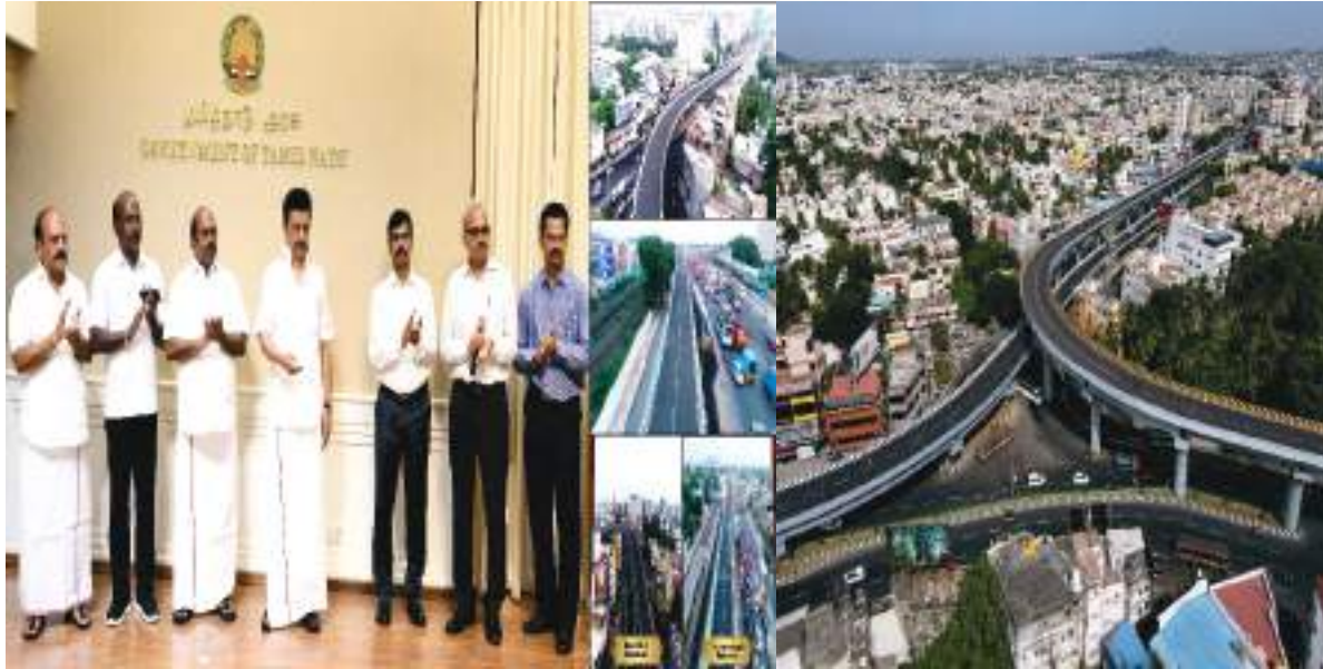
Grade Separator at Velacherry Vijayanagaram level -1 – Inaugurated by Hon'ble Chief Minister through Video Conference on 17.09.2022
