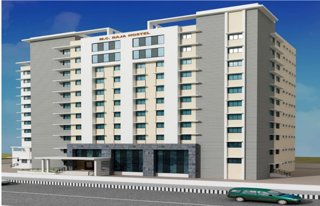
M.C.Rajah Hostel, Saidapet, Chennai-Front Elevation
